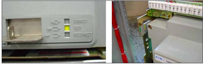
Figure 30. Switching Device in the TEST Position.
